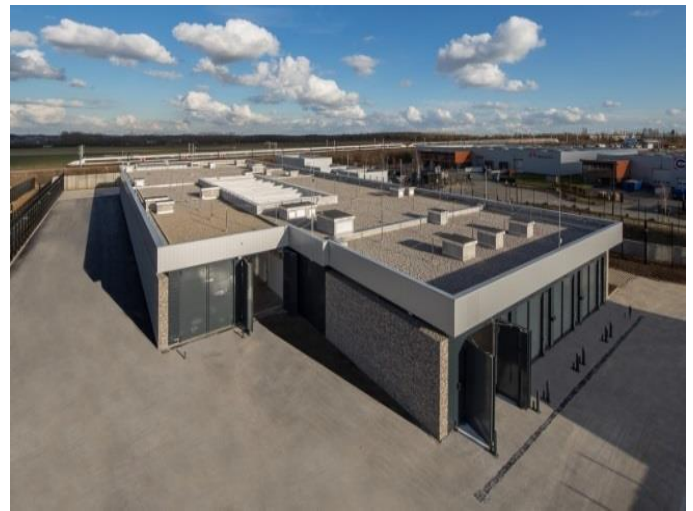
The cash management centre for the north of France (Cefinof), under construction close to Lille
